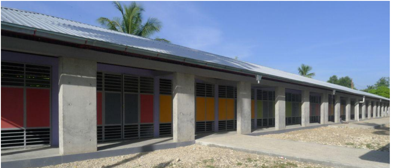
Main building with 9 classrooms in a row
