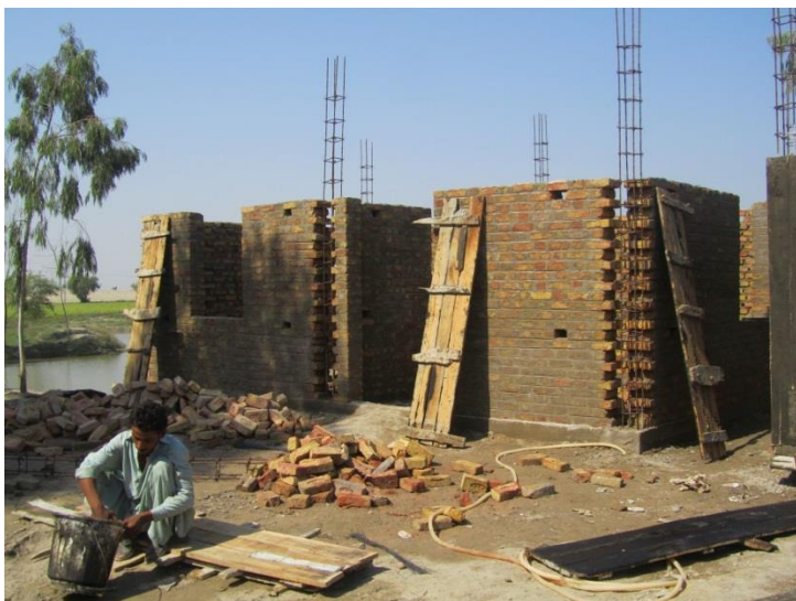
Confined masonry walls and reinforcement work.
