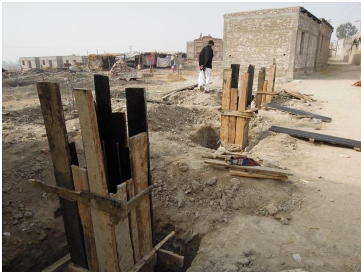
Installed formwork for the house foundations.
