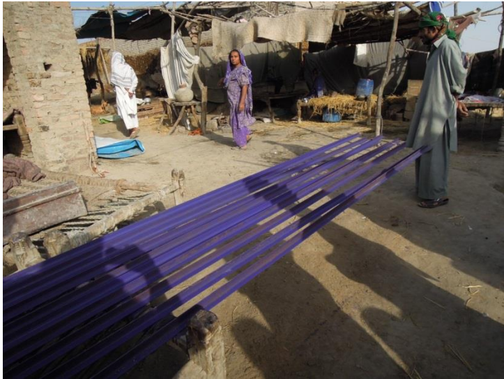
Cut and painted iron T-profiles for roof tile installation.
