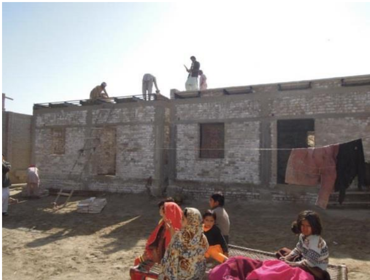
Ceiling and roof work.
