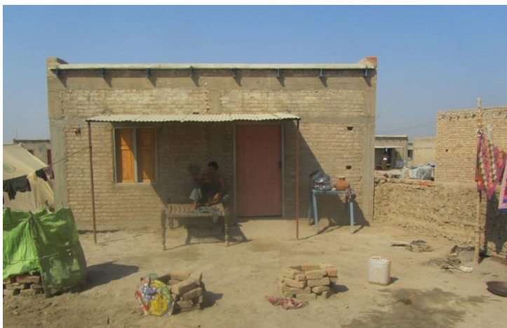
A completed house including planted tree and compound wall as part of the cultural environmental aspect.
