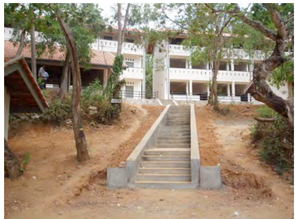
Main entrance to new 3 new buildings: H, L and K
