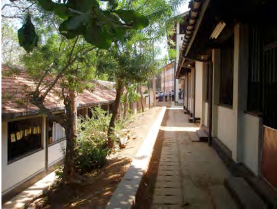
Renovated buildings I and J, E and F
