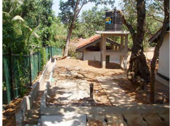
New toilets N and water tank ( 5000 lt)
