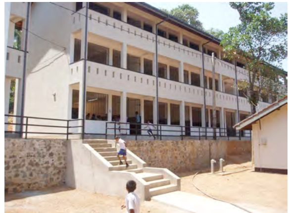
New building K with 15 classrooms
