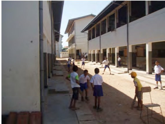
Building K and I with 14 renovated classrooms
