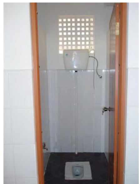
New toilet for students (E4 and E6)
