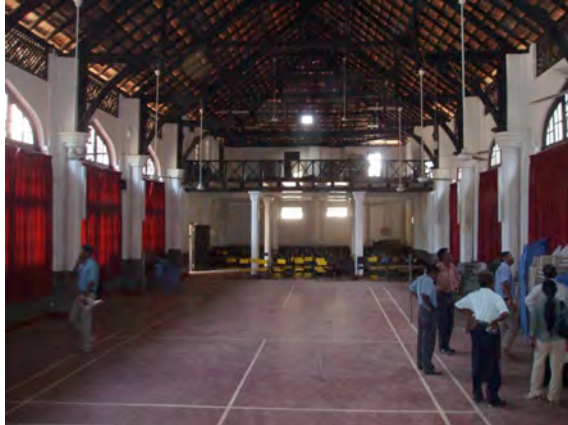
Auditorium (building C2) after renovation
