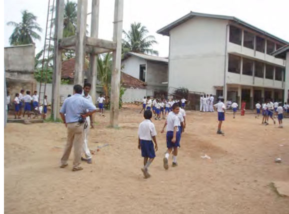
Playground, renovated building H and Water tower
