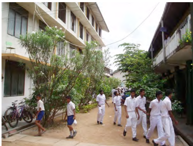
Entrance with building D: Principal, Computer room & classrooms
