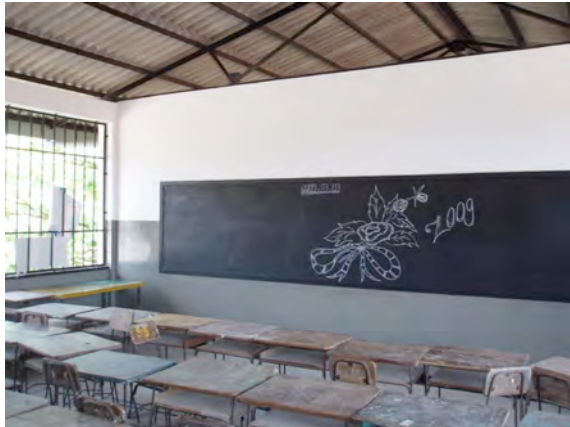
New renovated classroom in building H
