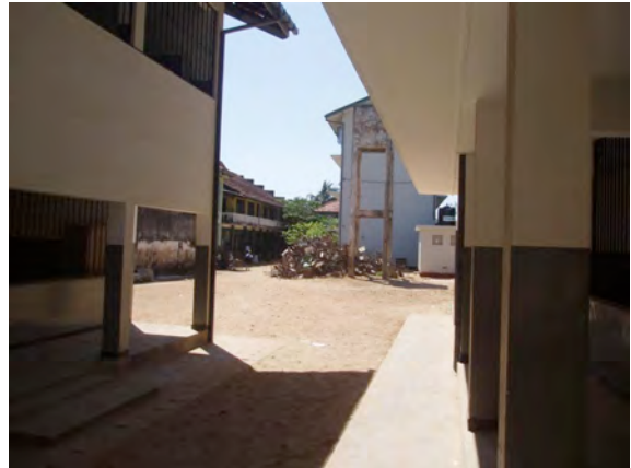
Building H and J with 14 renovated classrooms
