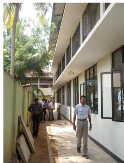
Renovated building N (backside)
