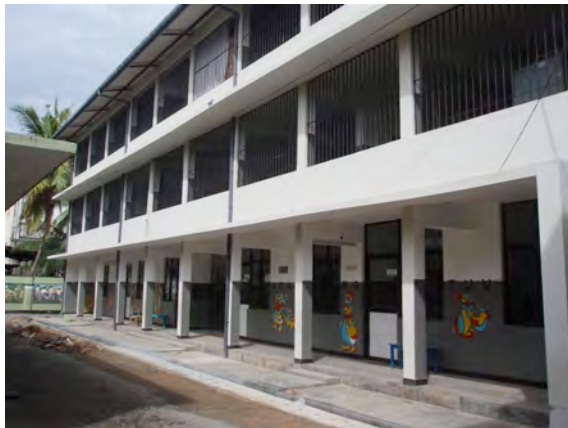
Building N (Primary) with 12 classrooms
