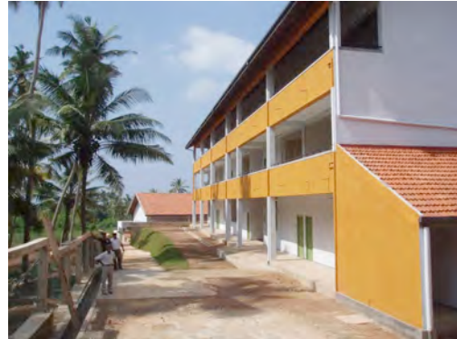
Ramp for disabled students to access A & toilet
