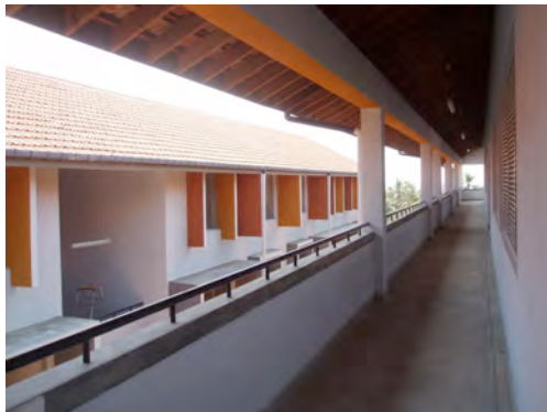
Building C: 12 class -, computer room & O/L Lab
