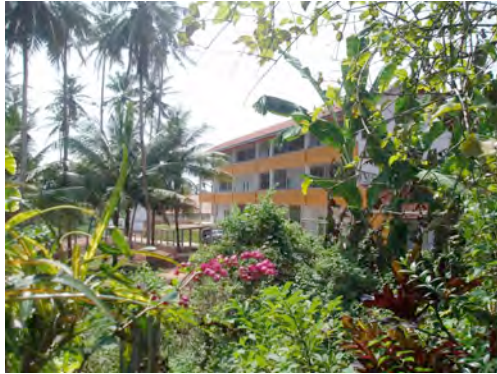
Building A: 13 class rooms and library
