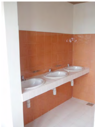
Building D: Male toilet
