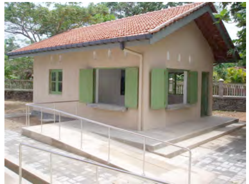
Building E: Canteen and kitchen
