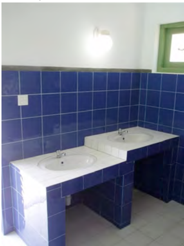
Building G: Male toilet
