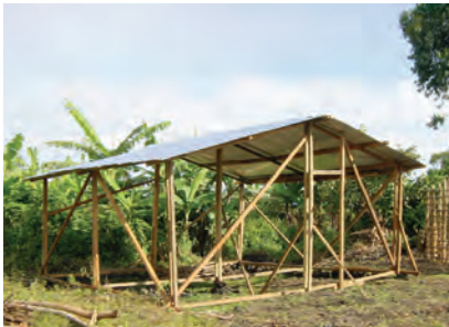
Structural skeleton of a house, showing cross-bracing
