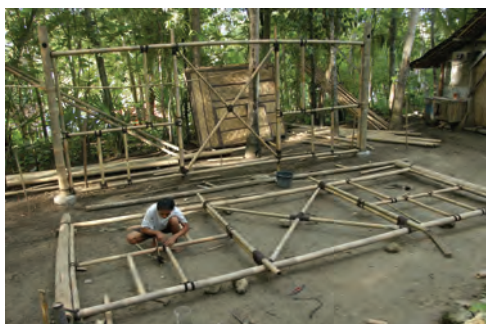
Prefabrication of a wall panel
