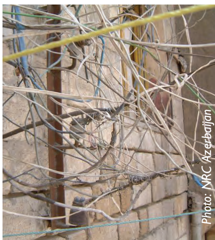
Wiring before upgrade
