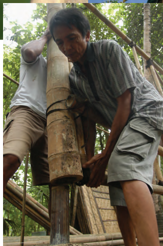
Connecting a vertical post to the foundation
