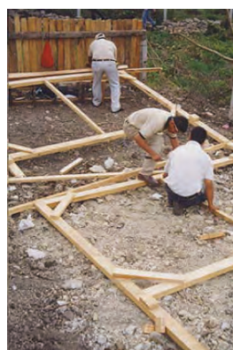
Prefabricating walls
