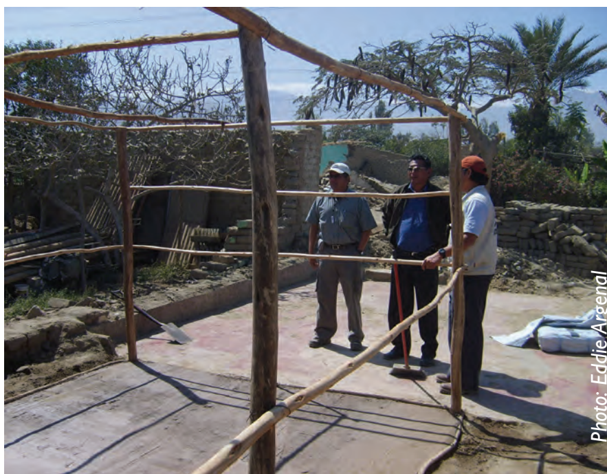
Round poles, not sawn timber, were used
