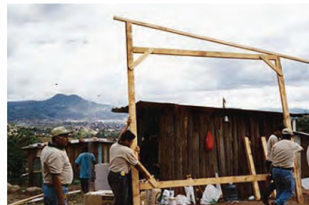
Shelter assembly using prefabricated walls
