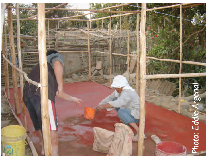
Making the concrete floor slab
