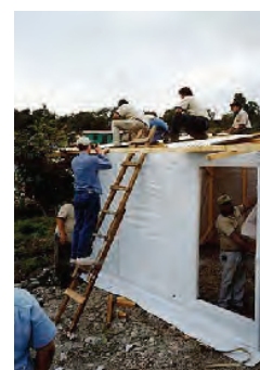
Covering the roof with corrugated iron
