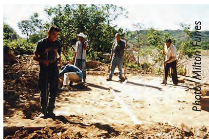
Marking out the site for a shelter
