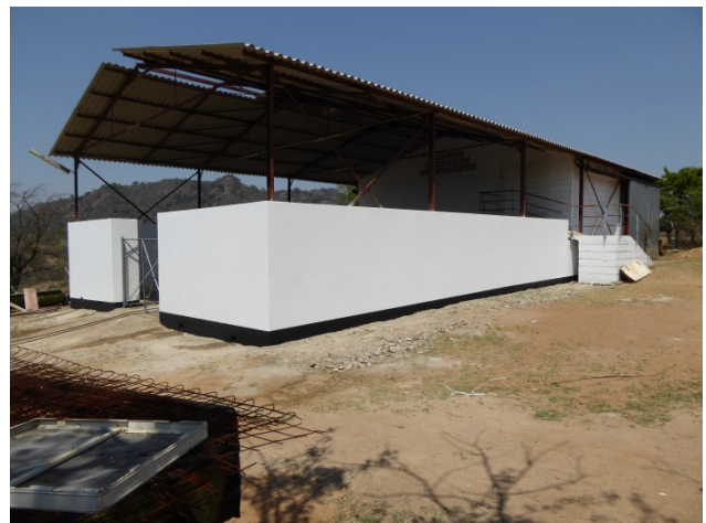
Weather enclosure Rupike (cranked ridge yet to be completed)
