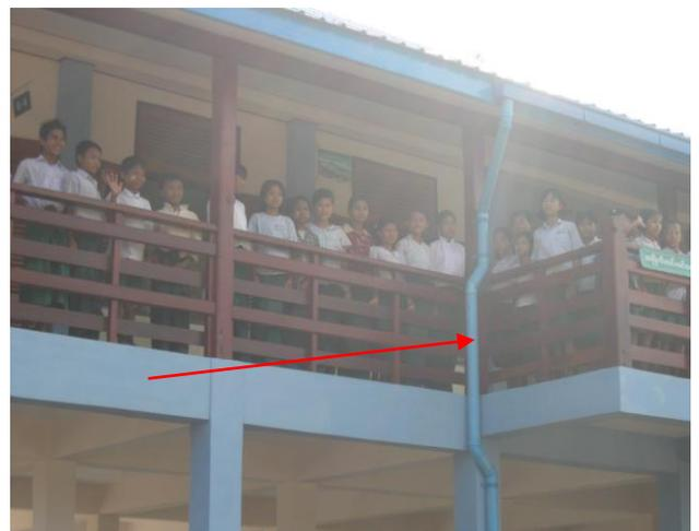
Complicated and expensive downpipe, not necessary, to be replaced by a simple outlet
