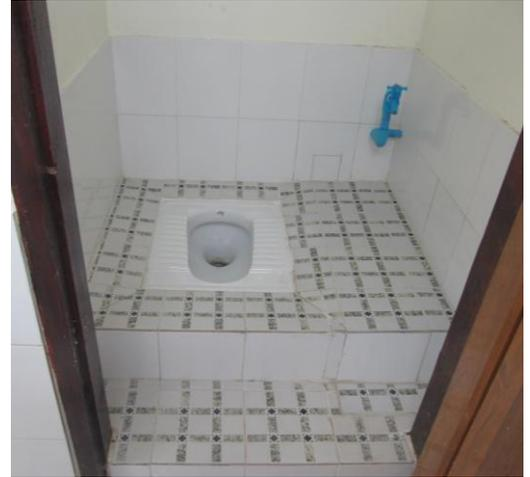
Appropriate floor pans flushed by bucket and fed with tap or shallow well
