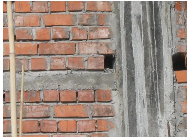
Correct connection between masonry reinforcement and column
