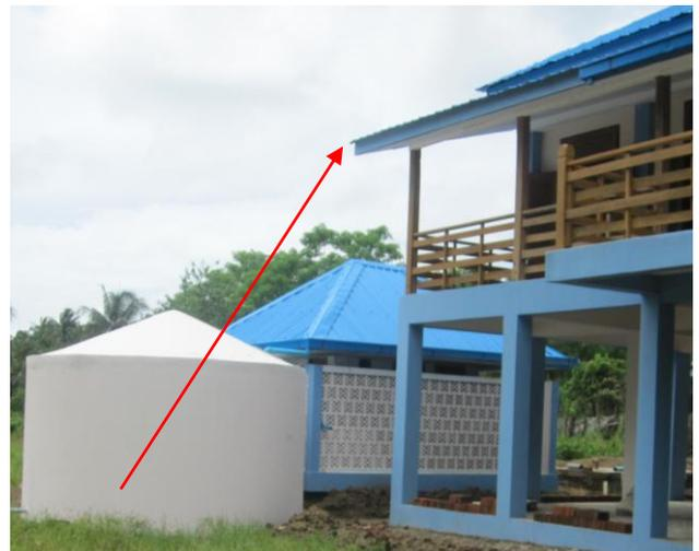
Wrong water source: the small toilet roof feeds the big water tank while the water of the main roof of the school is not utilized
