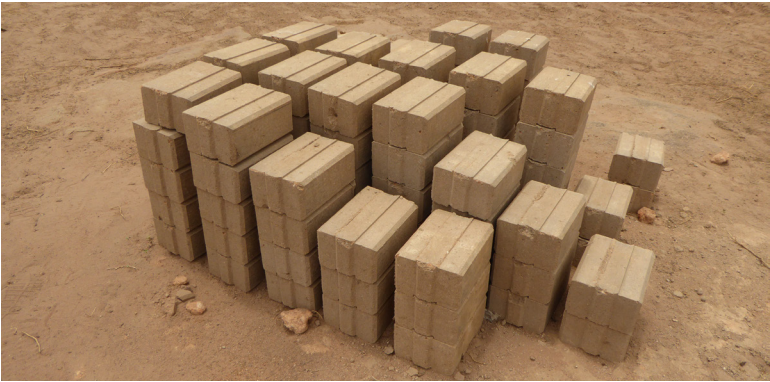
Produced on the site: ISS-Blocks after curing
