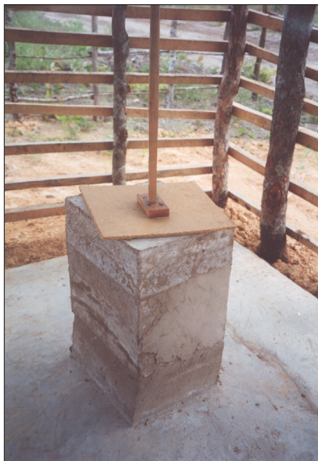
Sealed sharps pit, Zambia
