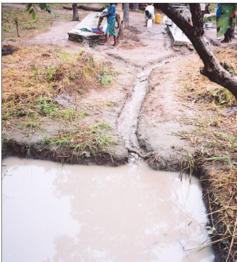
Poorly designed soakpit, Tanzania
