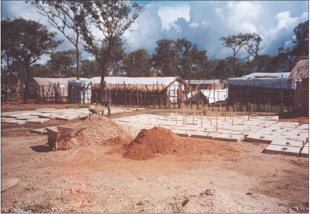
Preparation of concrete latrine slabs
