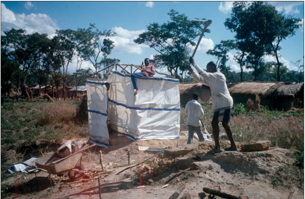
Pit latrine construction
