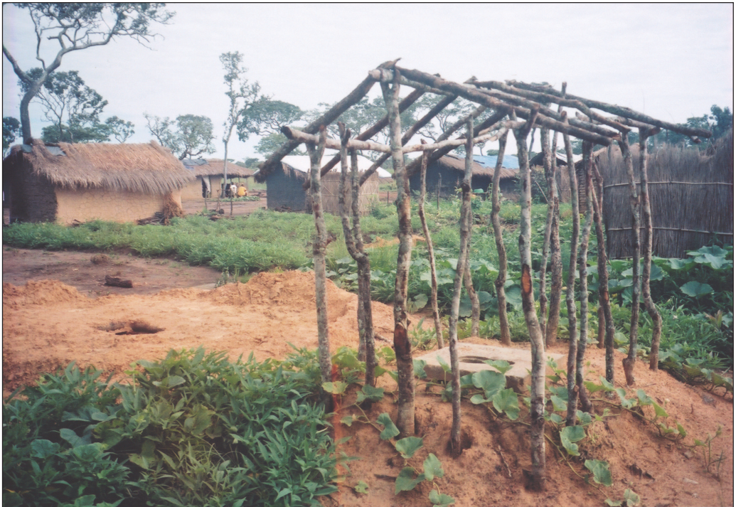
Family pit latrine under construction
