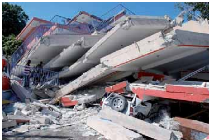
Earthquake damage in Haiti (2010)
