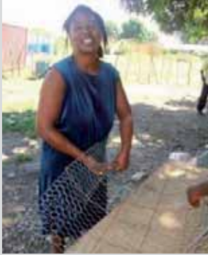
Preparing gabion cages IFRC
