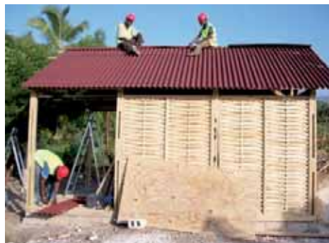
Production of infill panels for T Shelters in Haiti Handicap International
