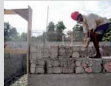
Forming gabion walls IFRC
