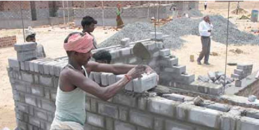
'Rat-trap bond' masonry Skat
