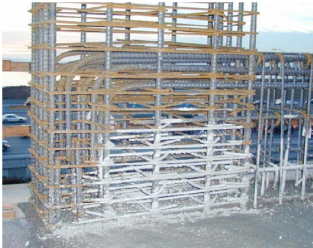
Figure 7-3 – Beam-column joint having multiple layers of beam reinforcement hooked at back side of joint. Note the upturned beam (the slab is cast at the bottom face of the moment frame beam).
