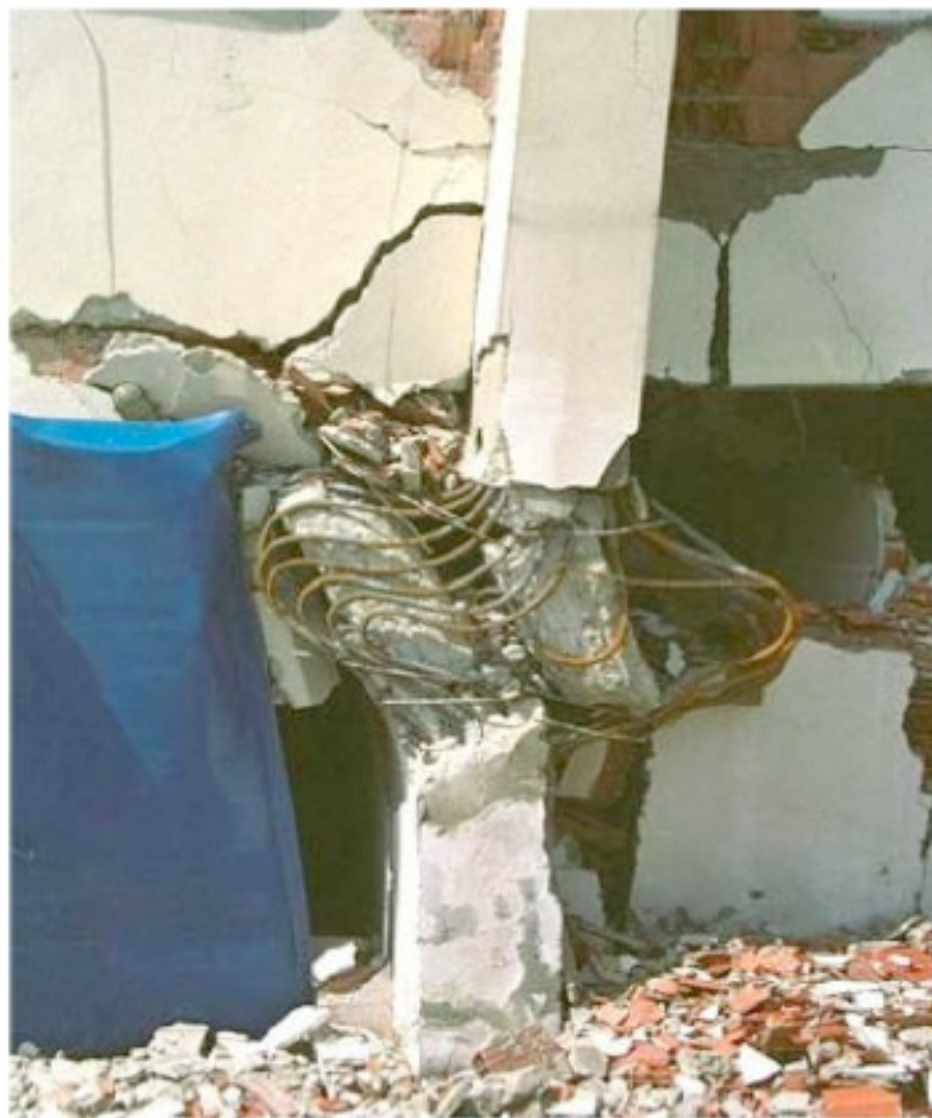
Figure 3-2 - Shear failure can lead to a story mechanism and axial collapse.
