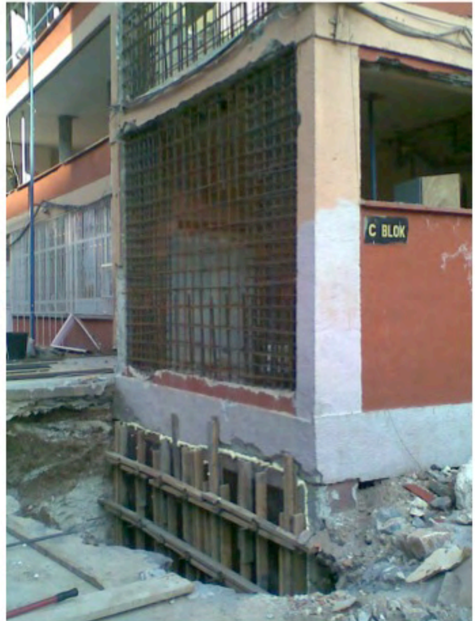
Retrofitting of a school at the Asian side
