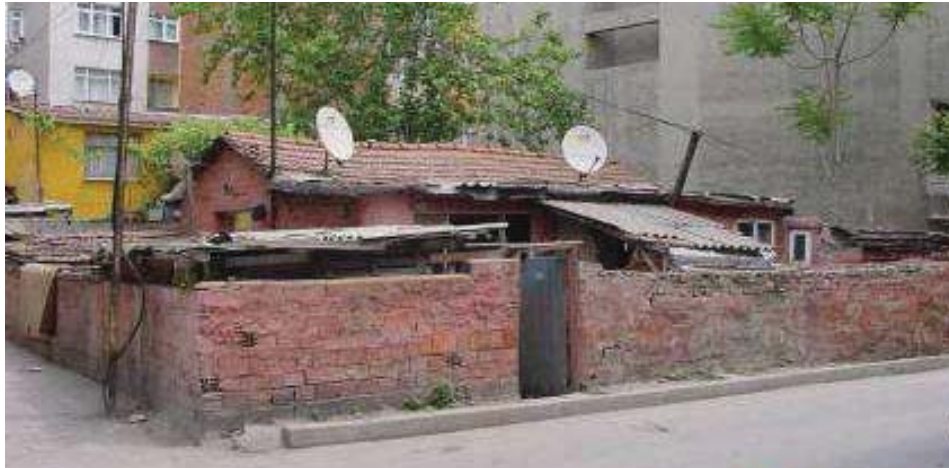
Image 21 : Constructed in 60's
