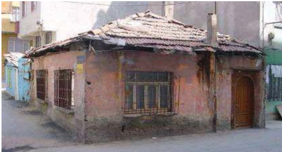
Image 22 : Constructed in 60's
