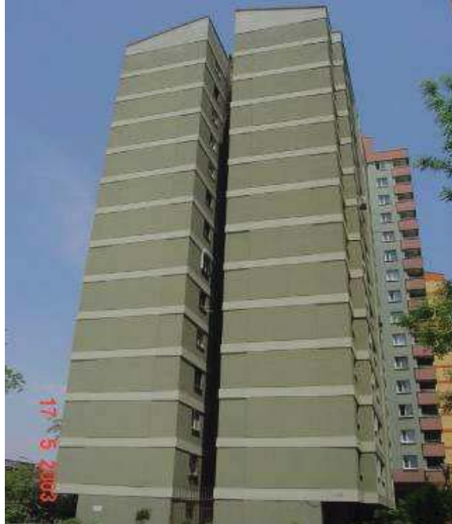
Image 26 : Constructed in 90's
