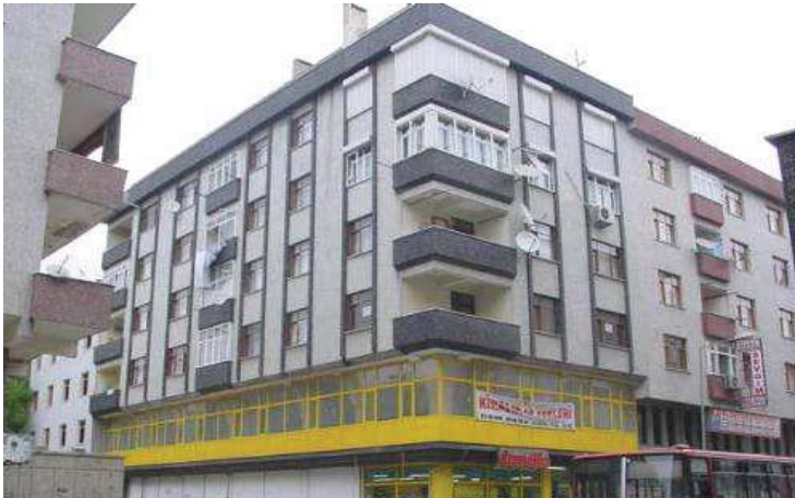
Image 24 : Constructed in 80's
