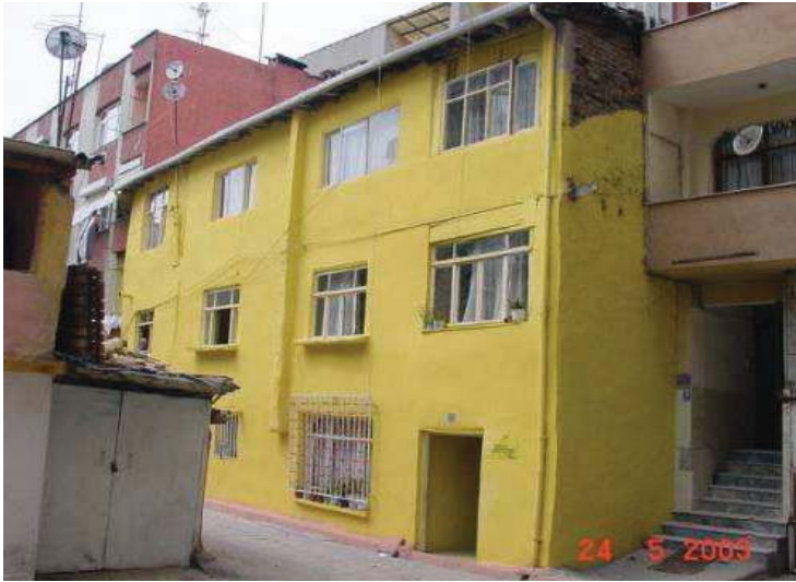
Image 23 : Constructed in 70's
