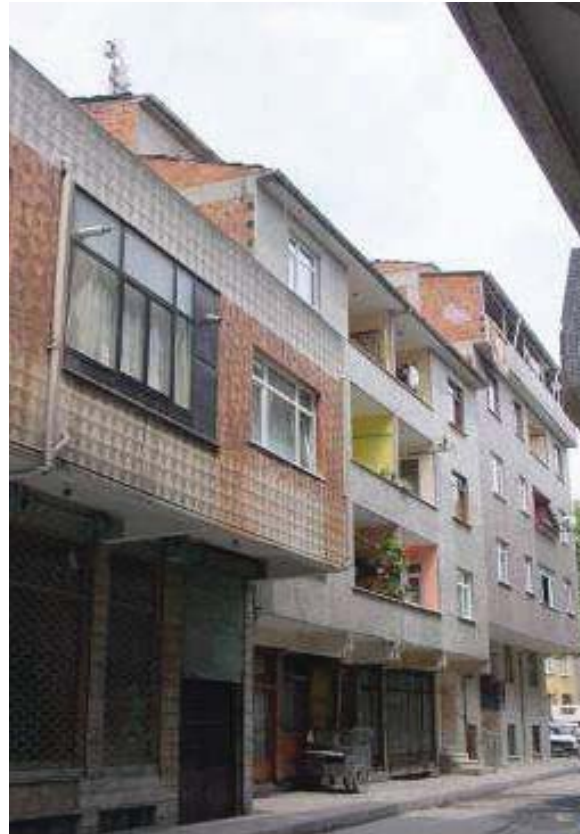
Image 25 : Constructed in 70's
