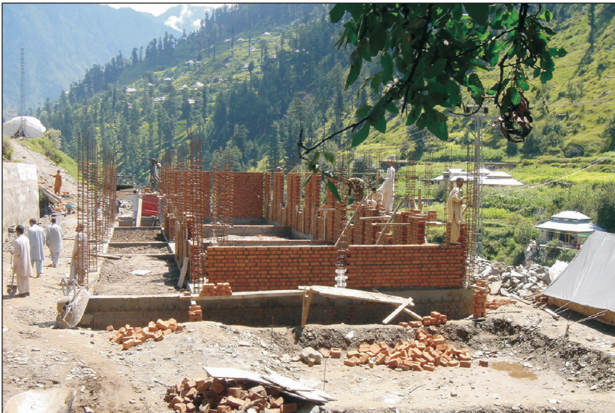
GPS Bari Maidan, brick wall construction
