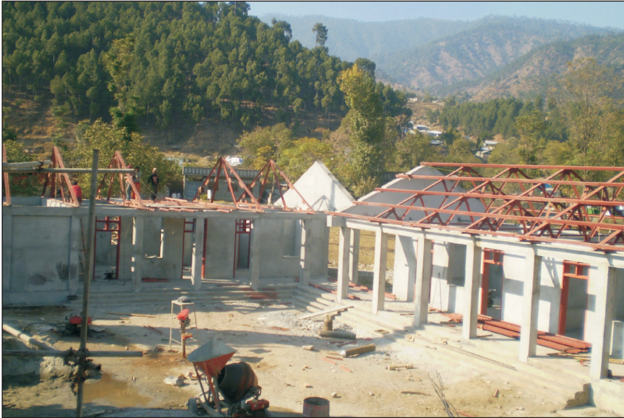
GPS Shohal Najaf Khan, steel roof truss erection
