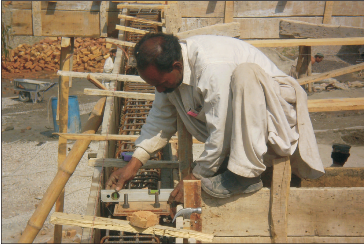
GGHS Charia, bond beam reinforcement work
