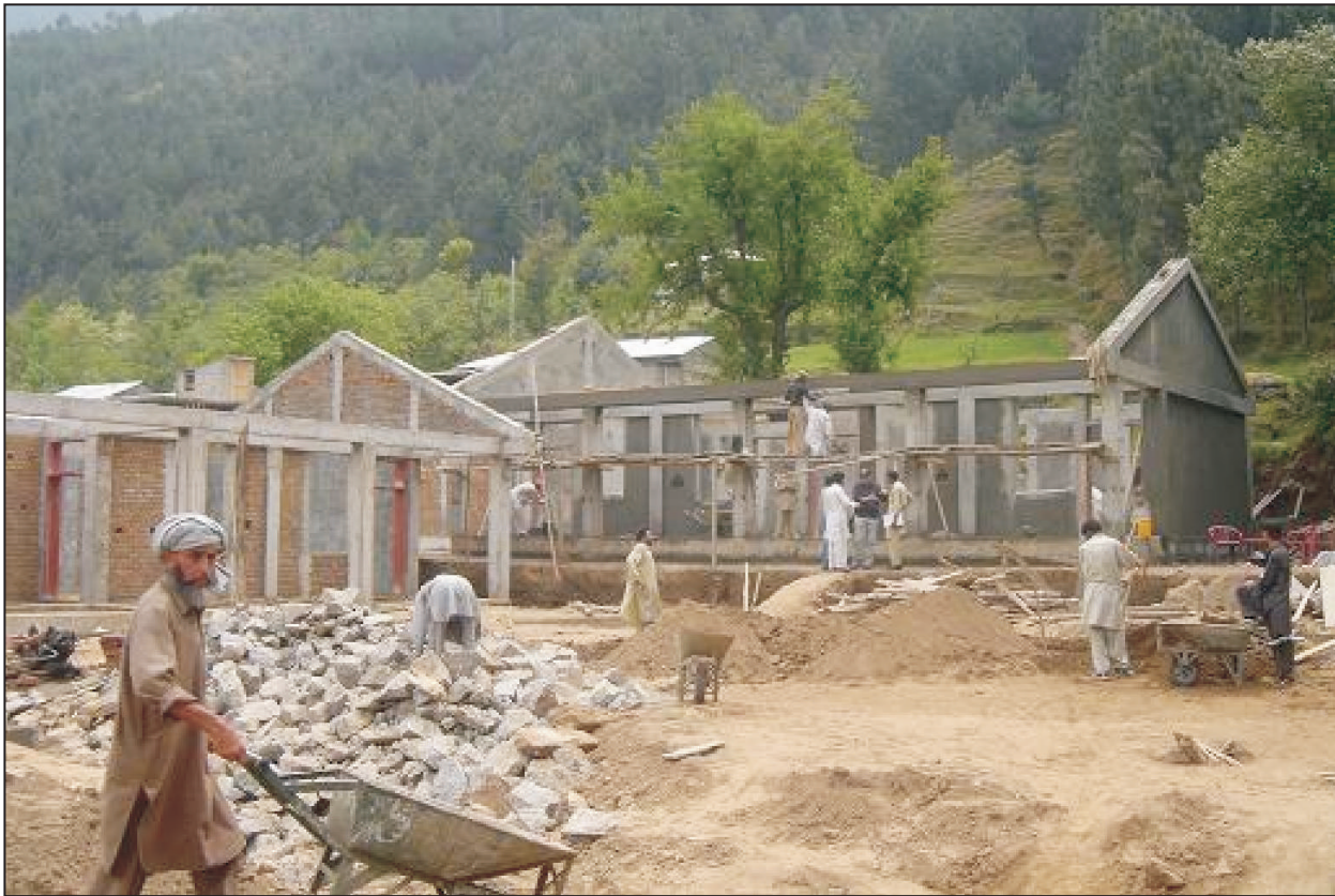
GPS Andrasi, plaster work
