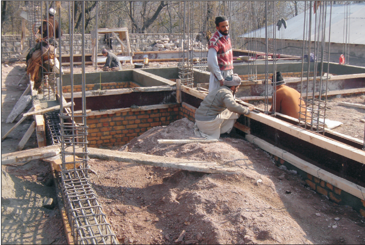
GGHS Talhatta, plinth beam construction
