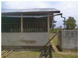
Result of poor roof gutter installation on a four years old school (not SDC built)
