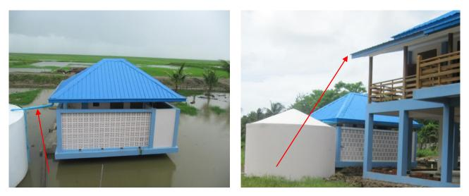
Wrong water source: the small toilet roof feeds the big water tank while the water of the main roof of the school is not utilized
