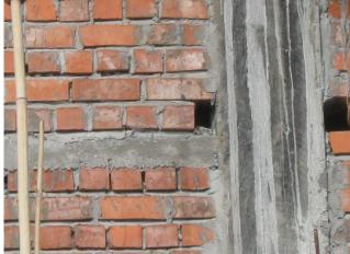
In some cases the masonry reinforcement beam not connected to column
