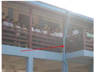
Complicated and expensive downpipe, not necessary, to be replaced by a simple outlet
