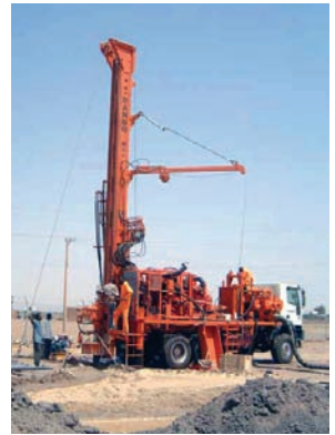
Figure 7: The Dando Watertec 24 drilling rig
