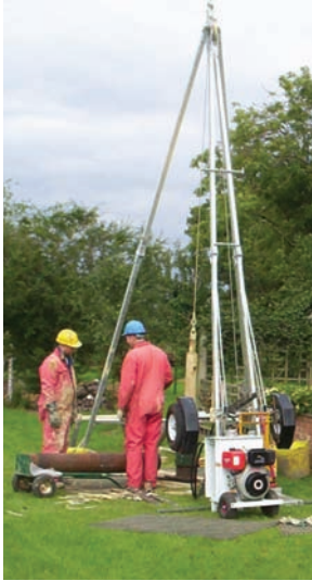
Figure 4: The Forager 55 cable-trailer rig in use
