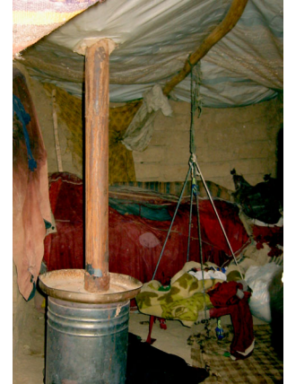
inside a self built shelter with adobe walls and plastic roof, , Maslack camp
