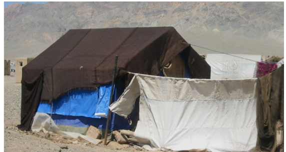
tent being insulated with the fabric from a Kuchi tent, Maslack march 2002
