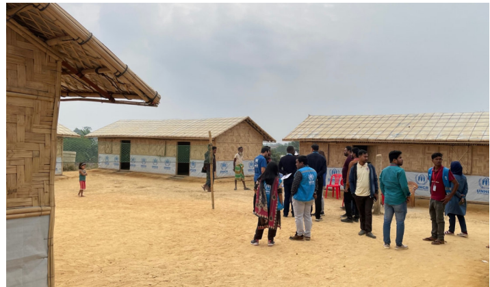
Pilot Camp 17 Shelters, built in steel pipes (Stilt Shelter)
