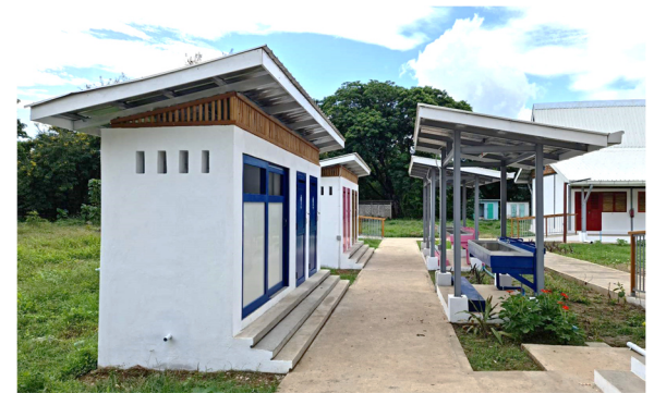
Toilet units for boys and girls with hand washing facilities
