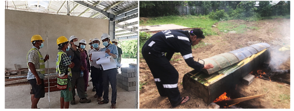
Architect visit construction site Bamboo treatment process
