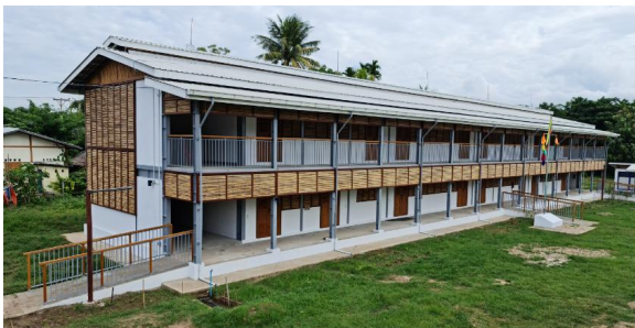
Two story steel structure building in Kon Khen Shan State
