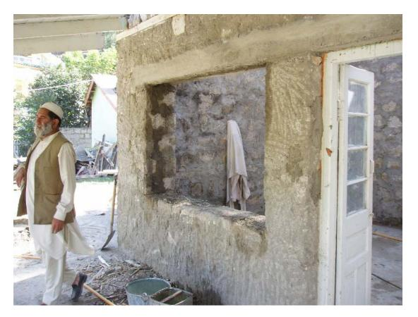
Replaced lintels above door and window
