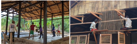
Temporary learning centre construction activities.
